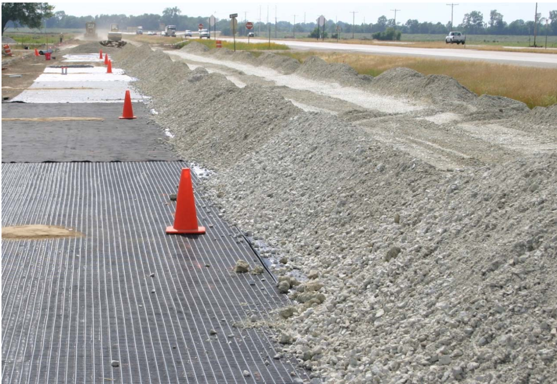
Figure 3.17. Base course placement on non-instrumented lane (Howard 2006).
