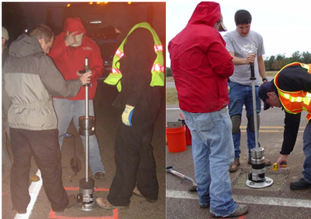
Figure 5.19. LWD tests conducted on asphalt and base course layers at Marked Tree site.
