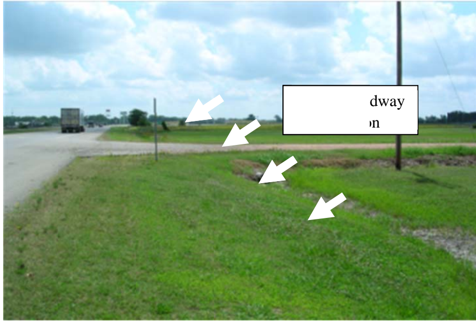
Figure 3.5. Test site prior to construction (Howard 2006).
