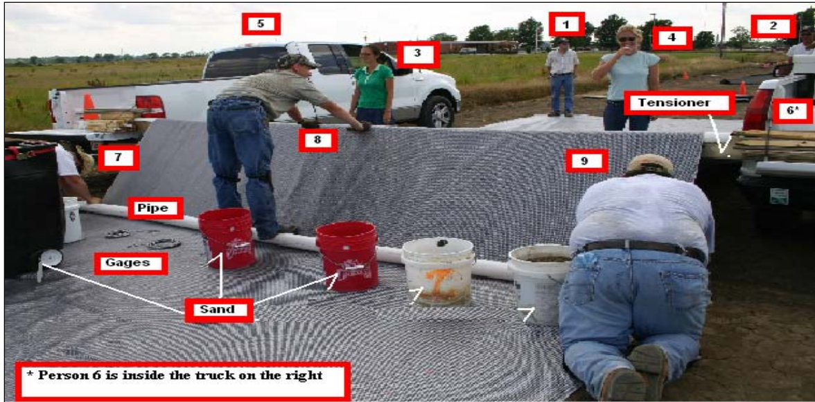
Figure 3.12. Geosynthetic tensioning technique (Howard 2006).
