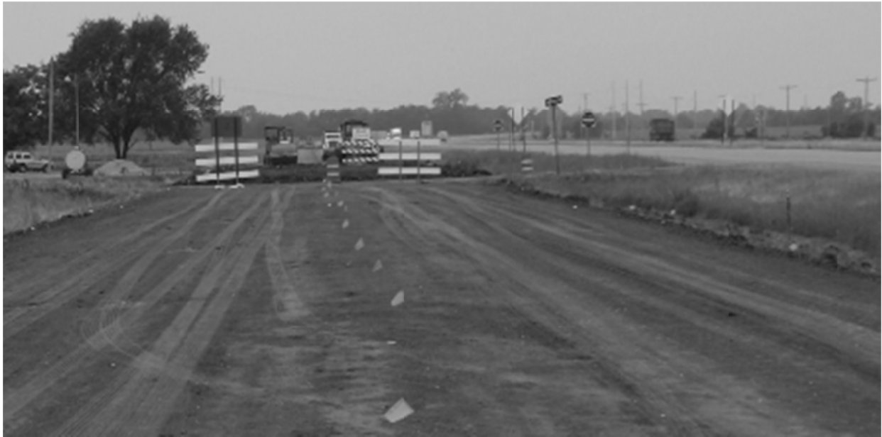
Figure 3.10. Finished cut subgrade (Howard 2006).
