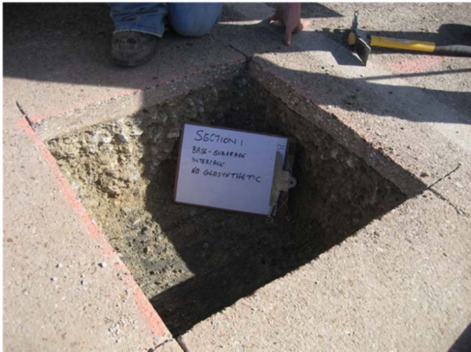
Figure 6.8. Base-subgrade interface of Section 1 (no geosynthetics).
