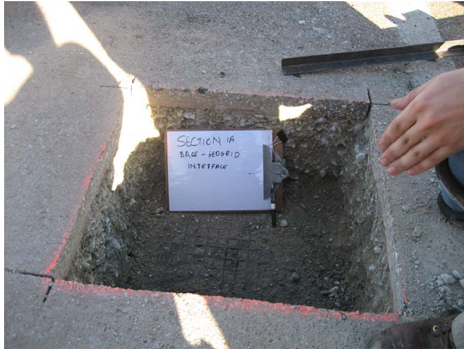
Figure 6.9. Subgrade-geosynthetic interface of Section 1A (Mirafi geogrid).
