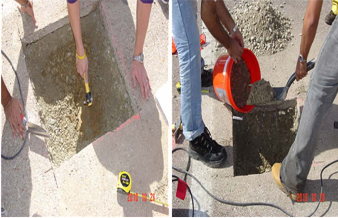
Figure 6.7. Base layer excavation and sampling at Section 2.
