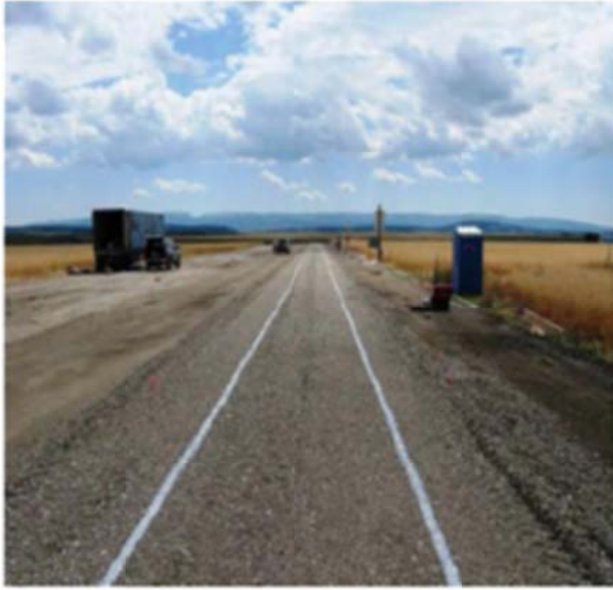
Figure 2.6. Full-scale field testing (Cuelho and Perkins 2009).
